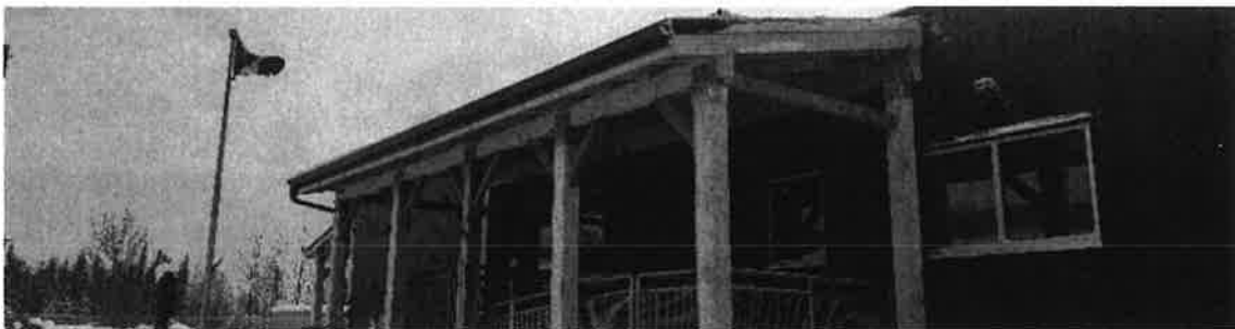
Faro Detachment (still under construction) nearing completion
