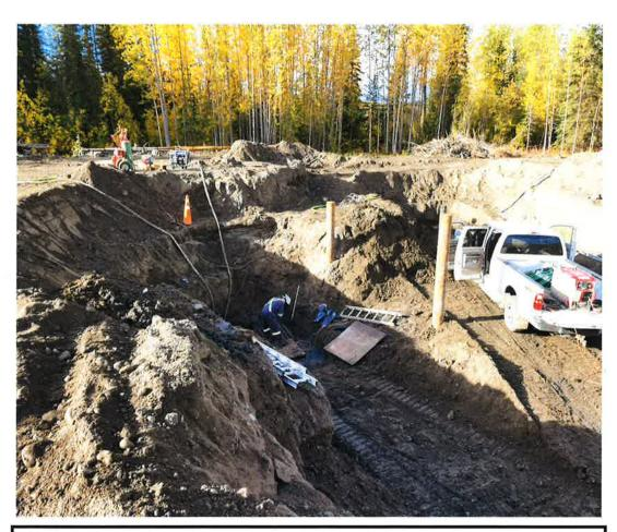
Faro Public Works employee Chris Wilkinson demonstrated his welding skills during the installation of new Water Well #6. He was standing on pallets because he was so close to the water table. The two pipes to the left of Chris were remnants of decommissioned wells from 2017. When the area is backfilled and brought back to grade, the ground level will be about 6' above the truck roof.
